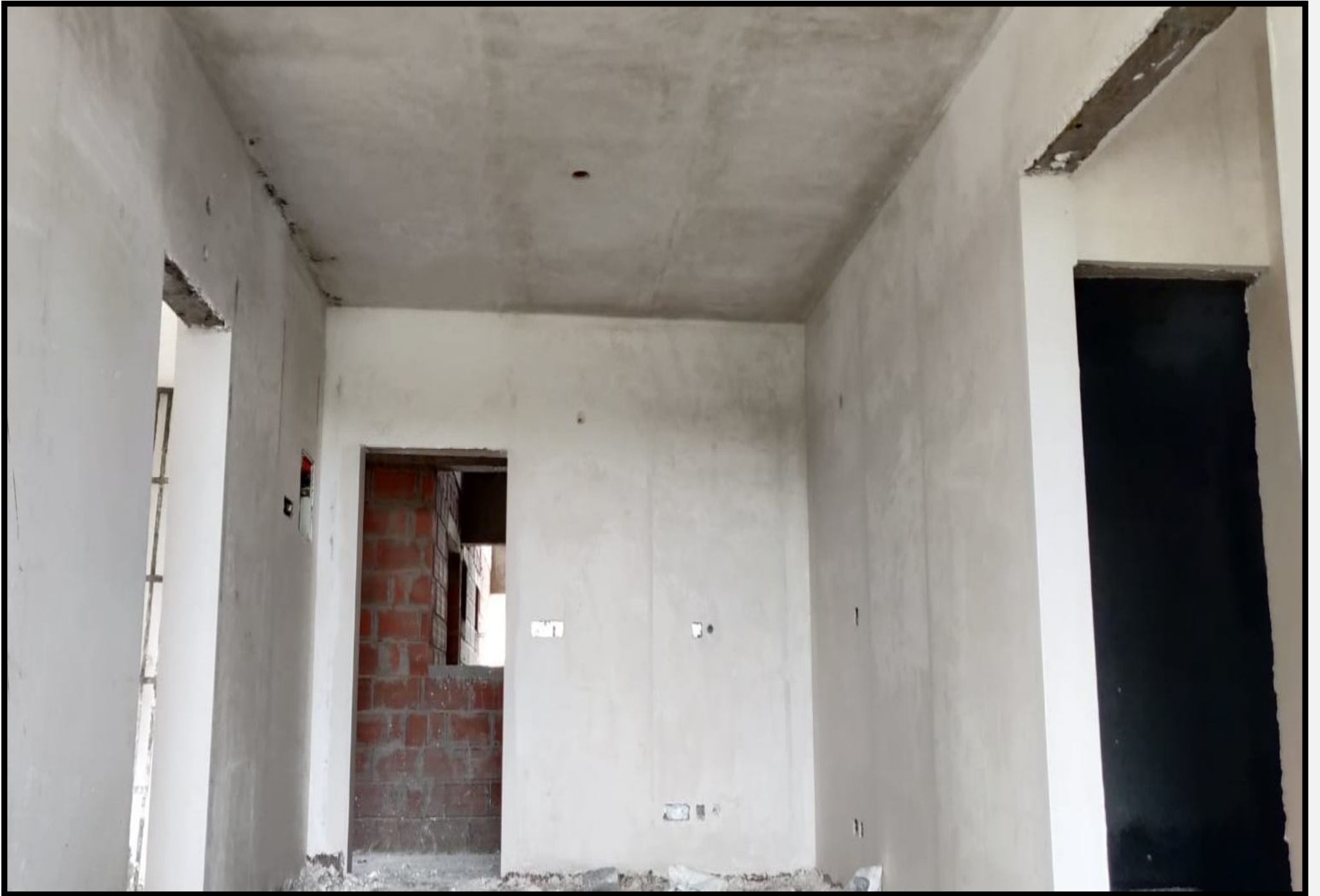
Internal plastering works
