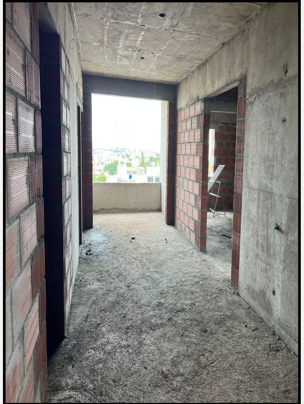
Block masonry works
