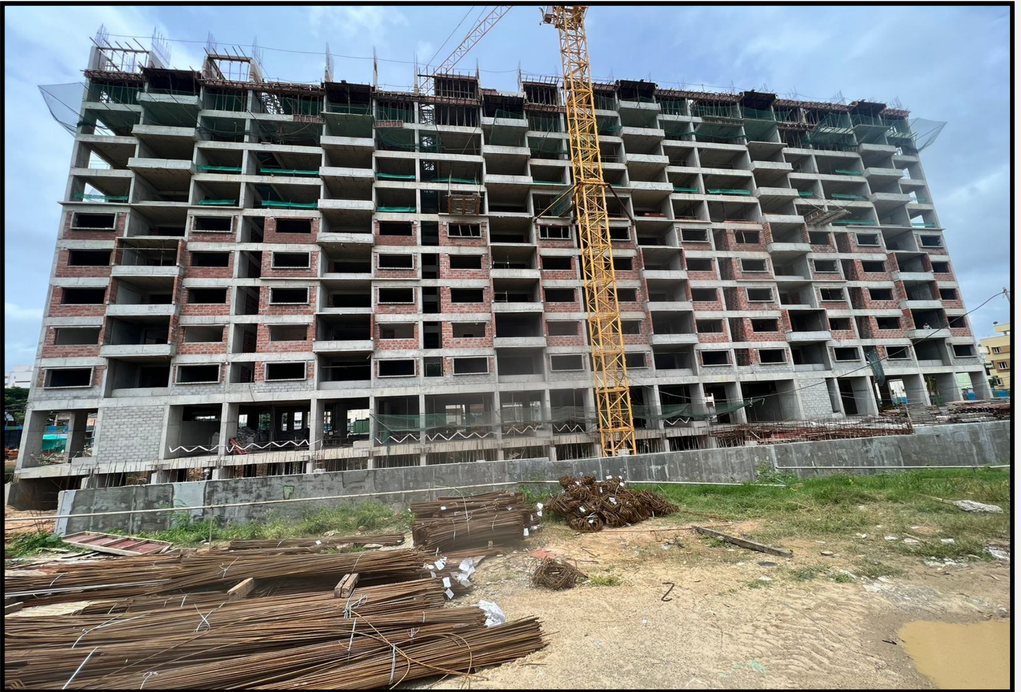
TOWER-01&02 VIEW FROM WEST FACE
