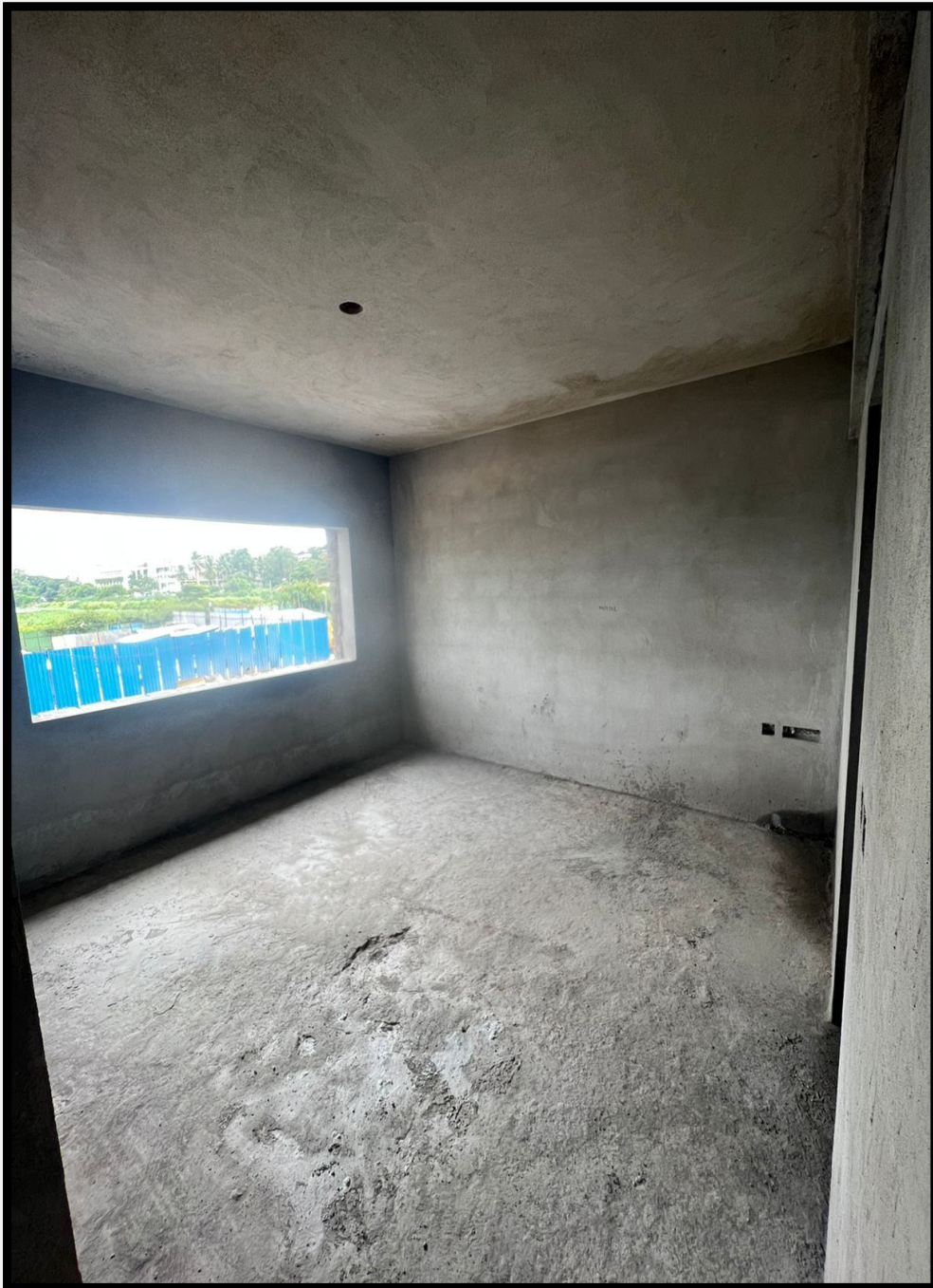
Internal plastering works
