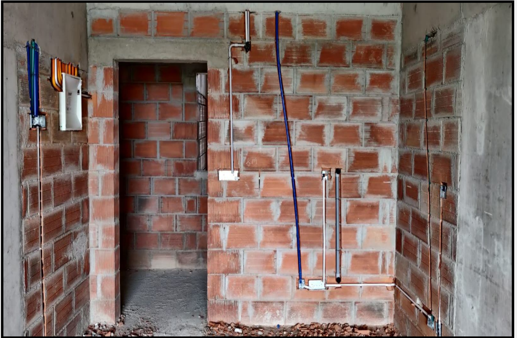
Electrical wall conduiting & GI box fixing works
