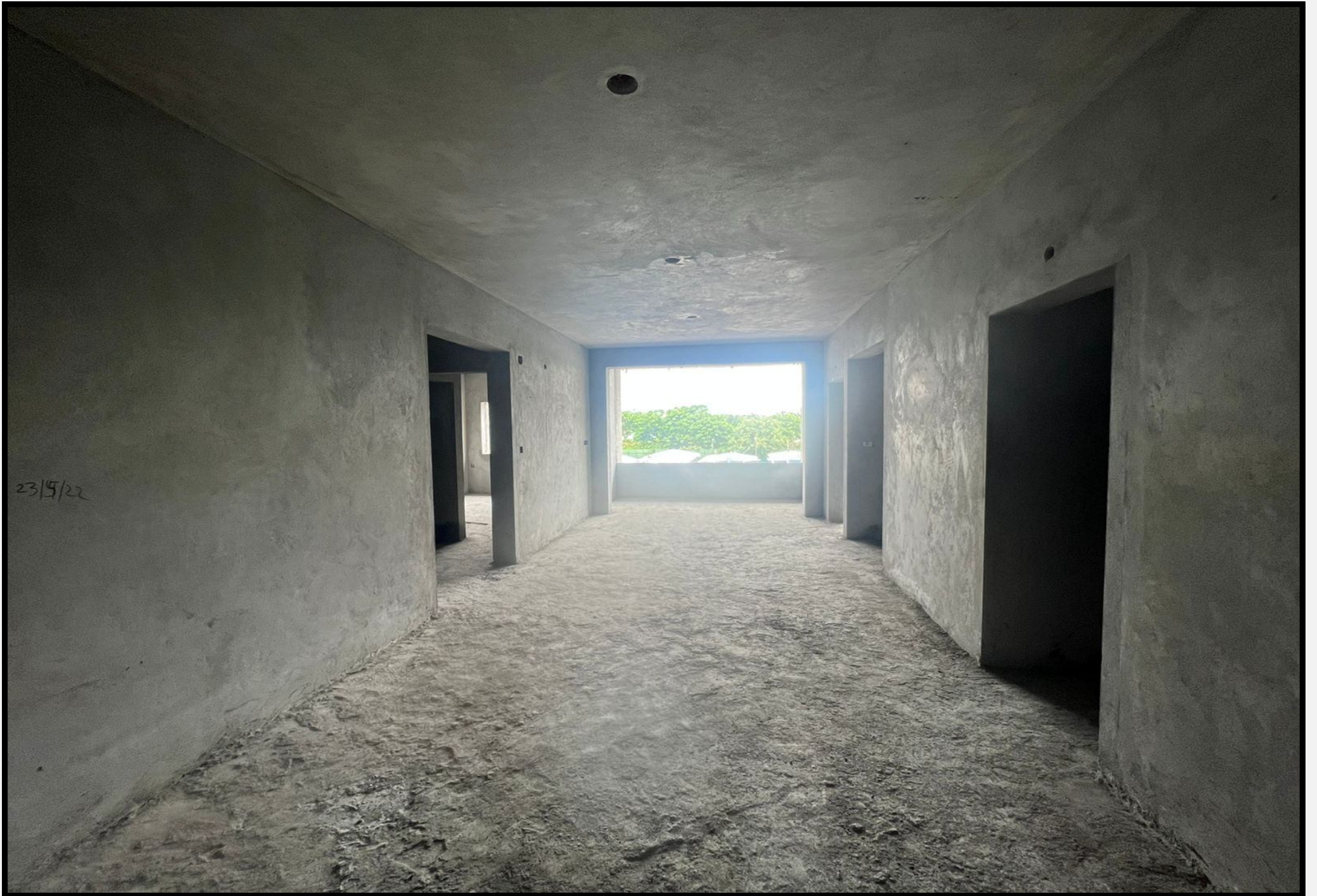
Internal plastering works
