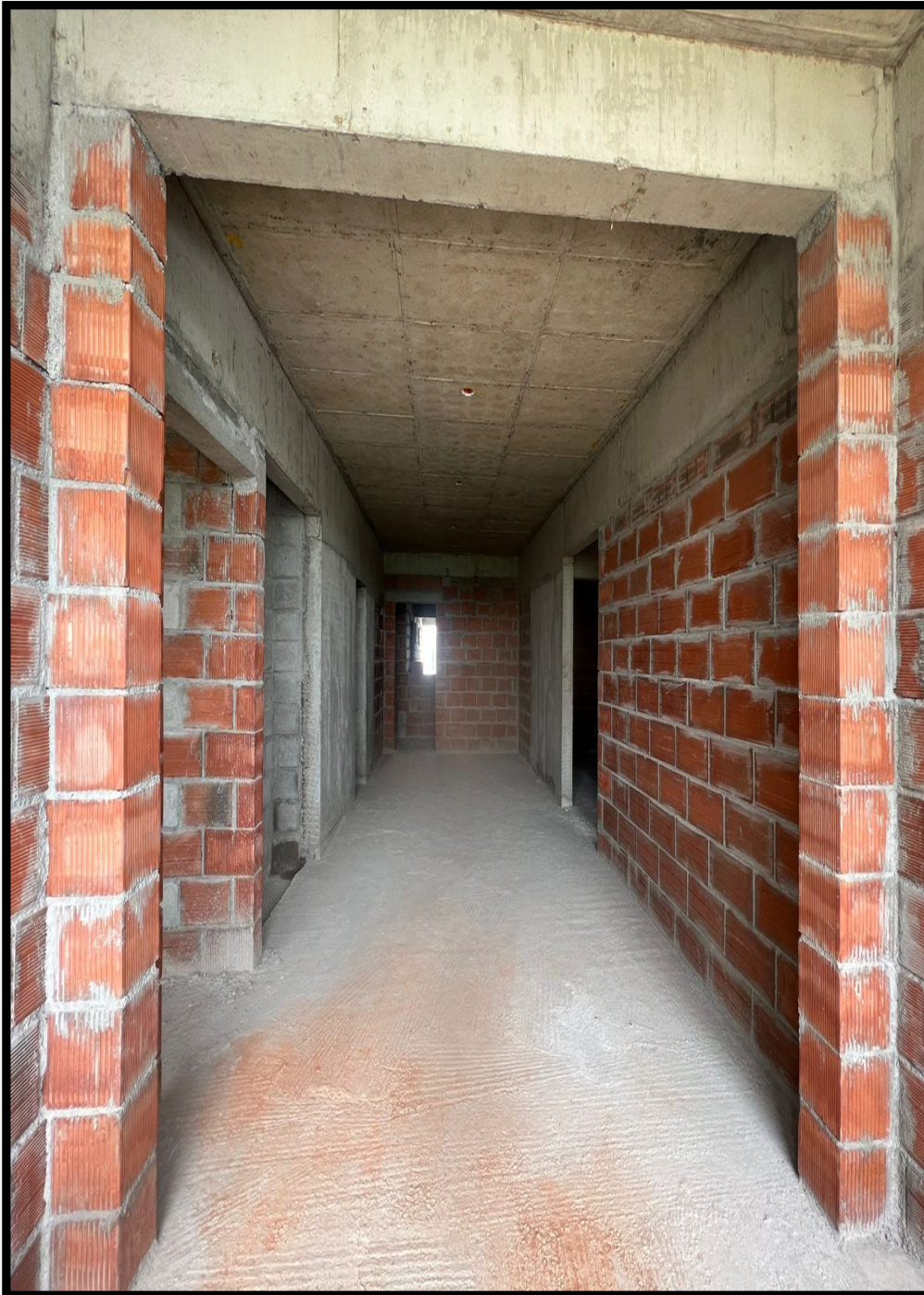
Block masonry works.
