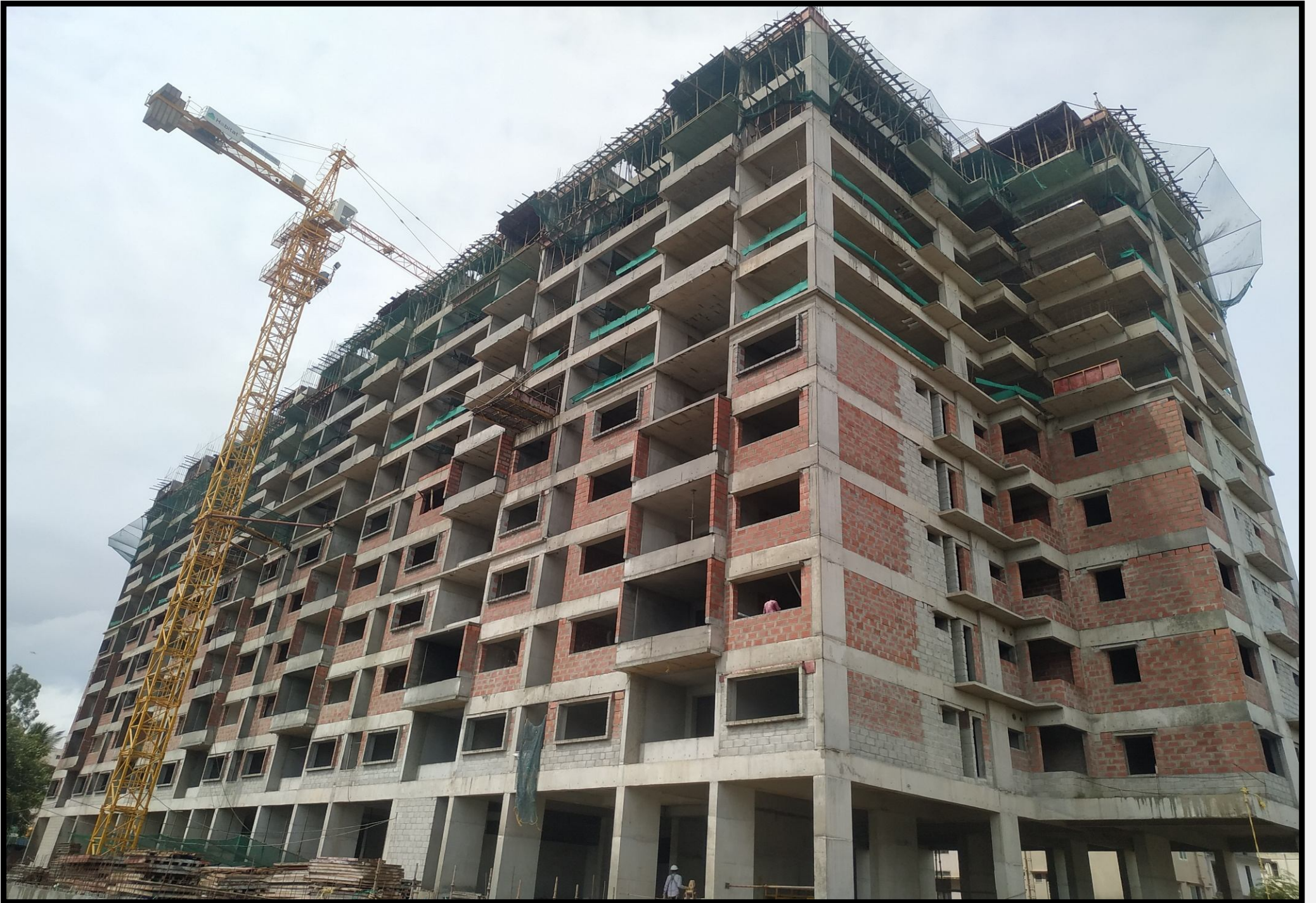
TOWER-01&02 VIEW FROM SW FACE
