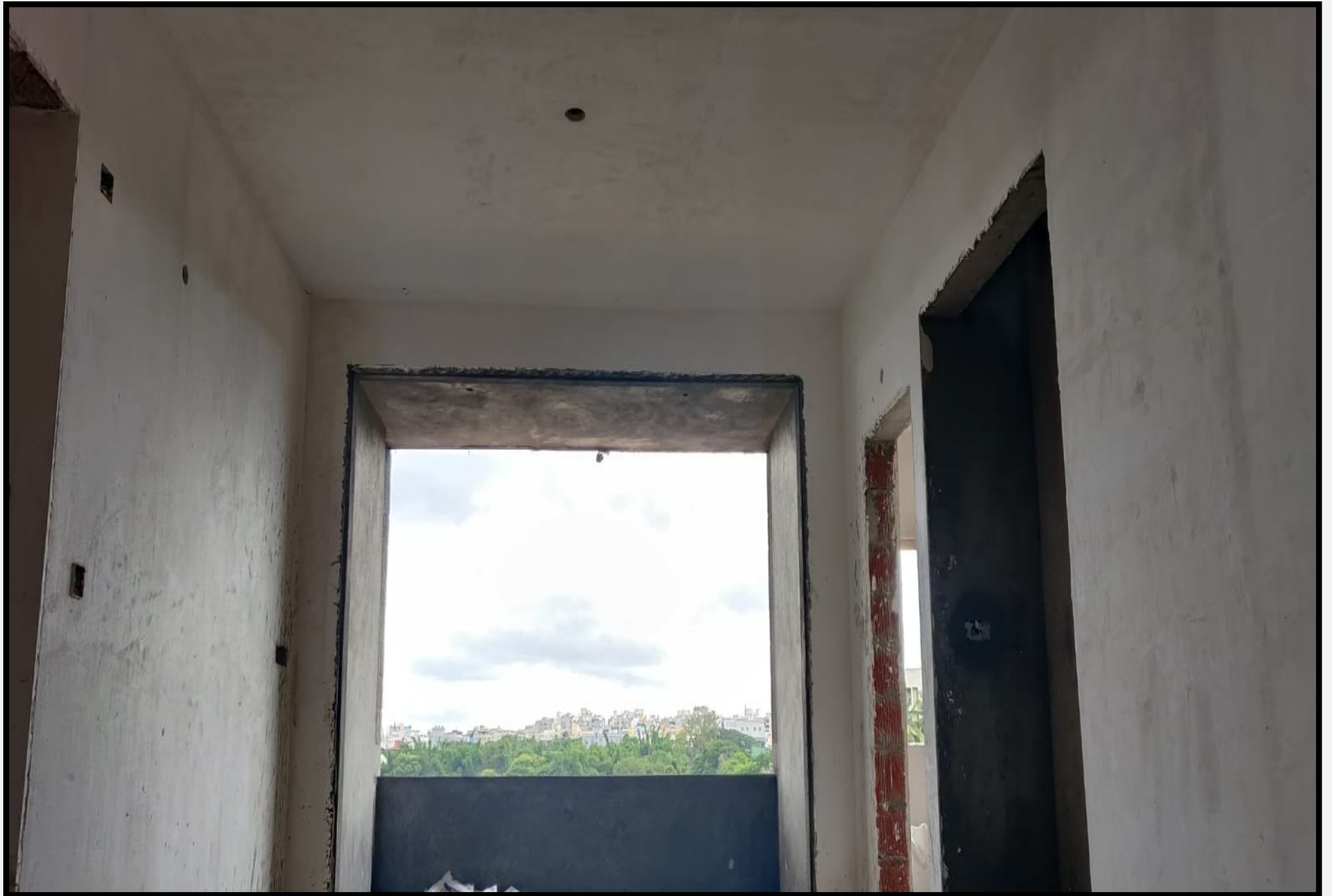
Internal plastering works
