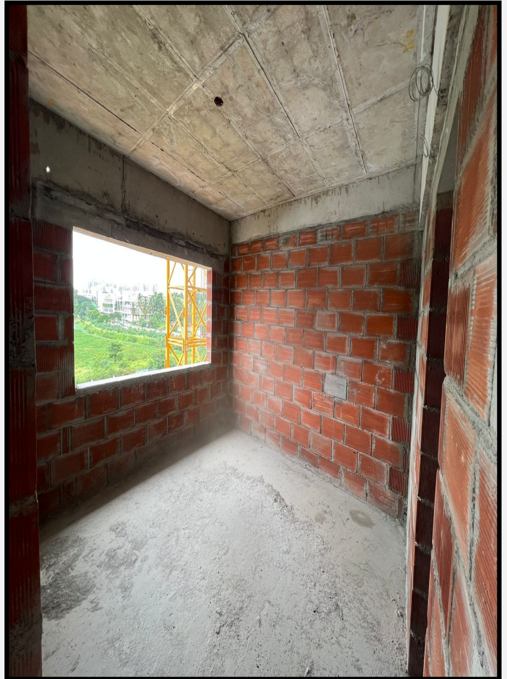
Block masonry works.
