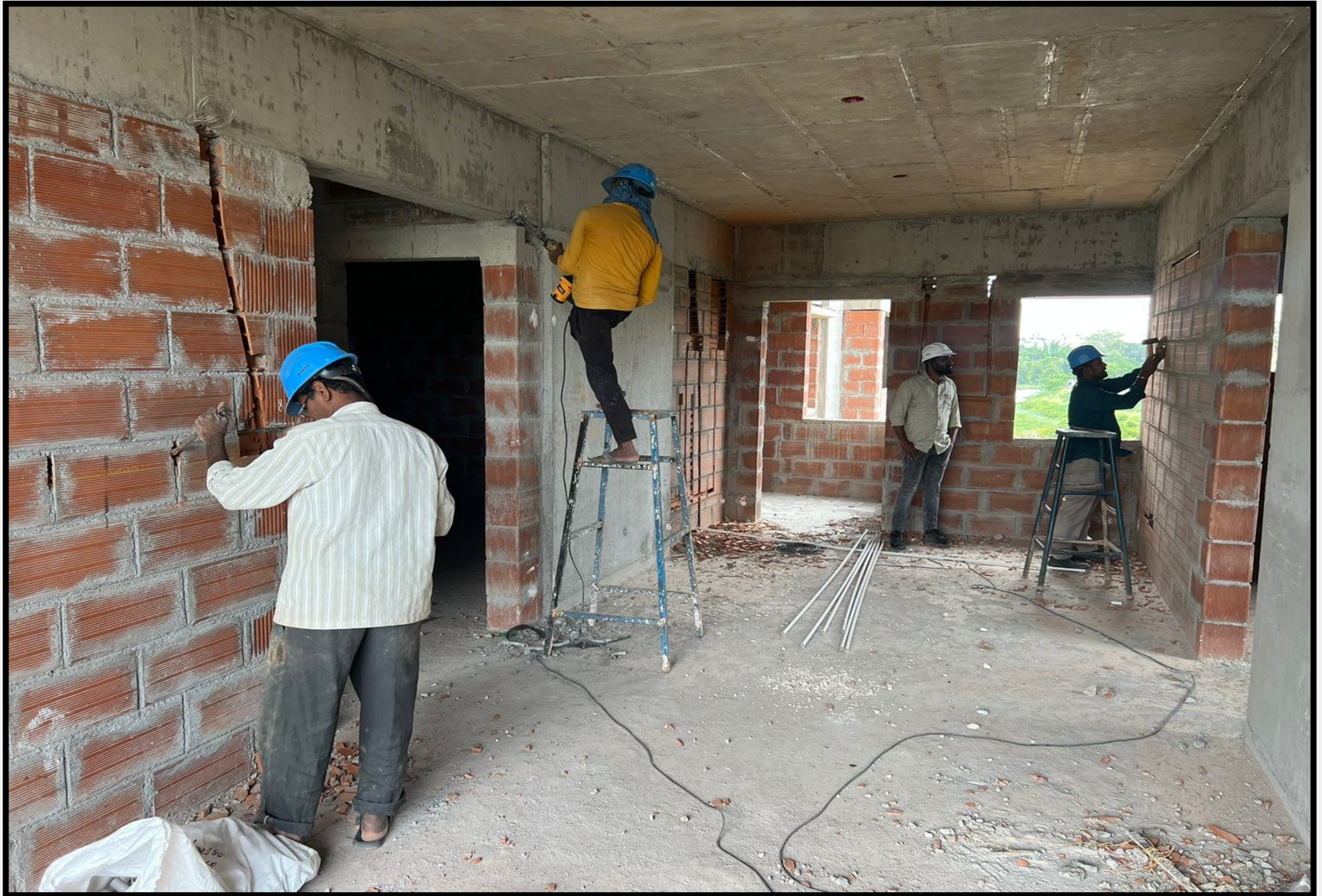
electrical wall conduiting & GI box fixing works
