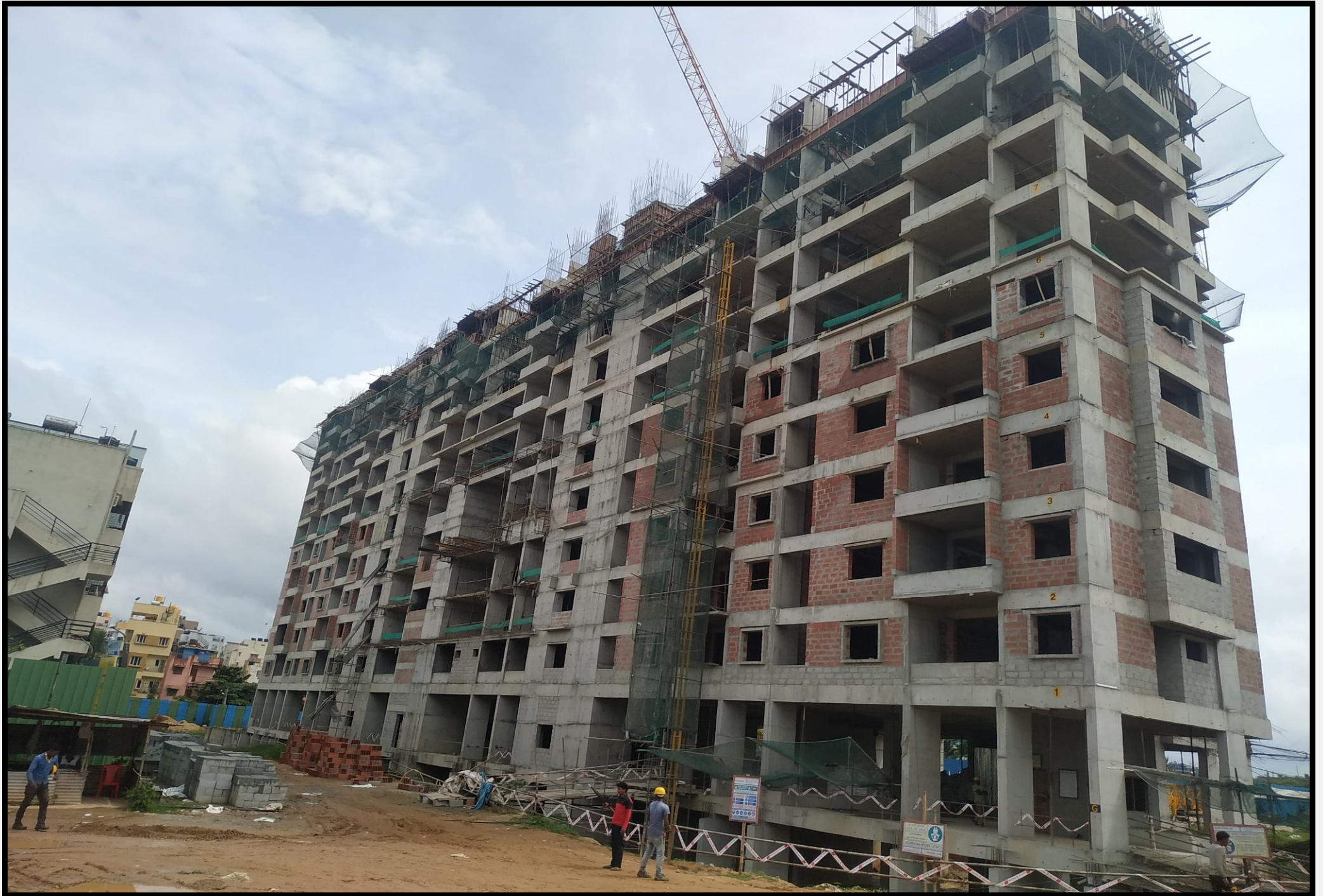
TOWER-01&02VIEW FROM NORTH EAST FACE
